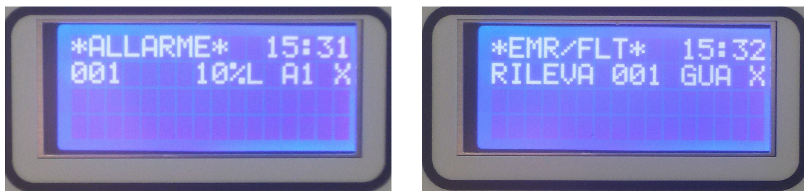
Figure 29 Active Events screen with Alarm and Fault
