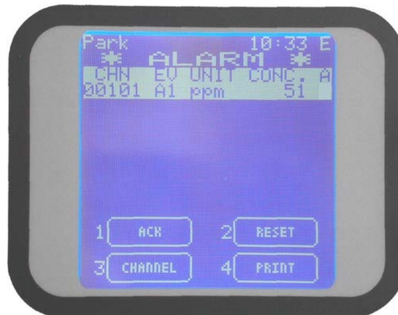
Figure 20 Typical ALARM state of the ACTIVE EVENTS screen.
